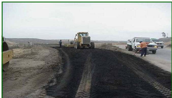
Spreading an Asphalt Mix Made with Recycled Asphalt Shingles (from www.shinglerecycling.org )
