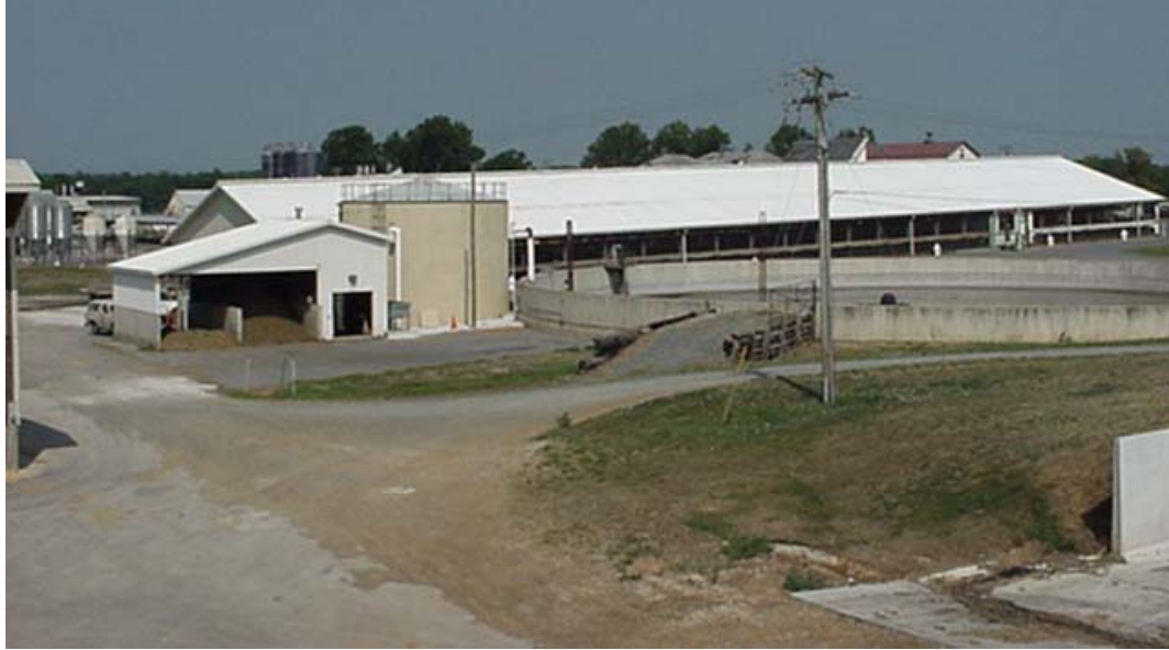
Figure 7-6 Dairy Manure Digester
