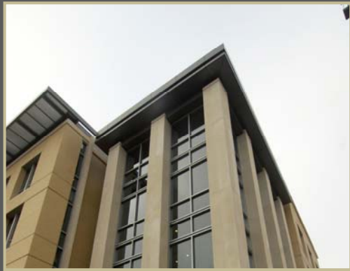
USC's Horizon Research Facility
