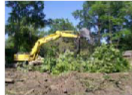
LCR offers land clearing services to its customers
