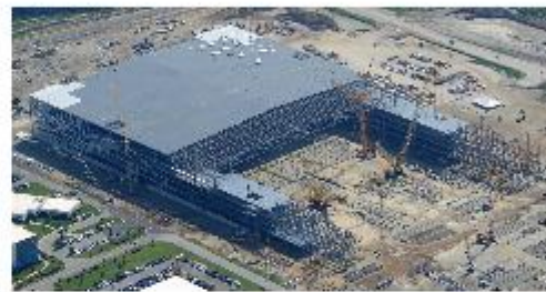
Boeing Project in Charleston, SC made with CMC steel
