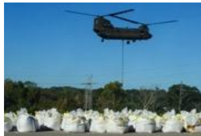
100 one-ton sandbags and equipment sling-loaded to the Columbia Canal.
