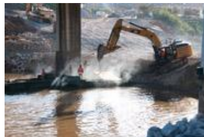
Engineer assets and construction support provided to the Columbia Canal project.
