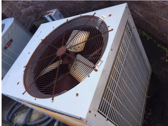
HVAC System at Waccamaw MHC 25 years old and original to the building. Need to be replaced due to age and environmental issues (salt air).
