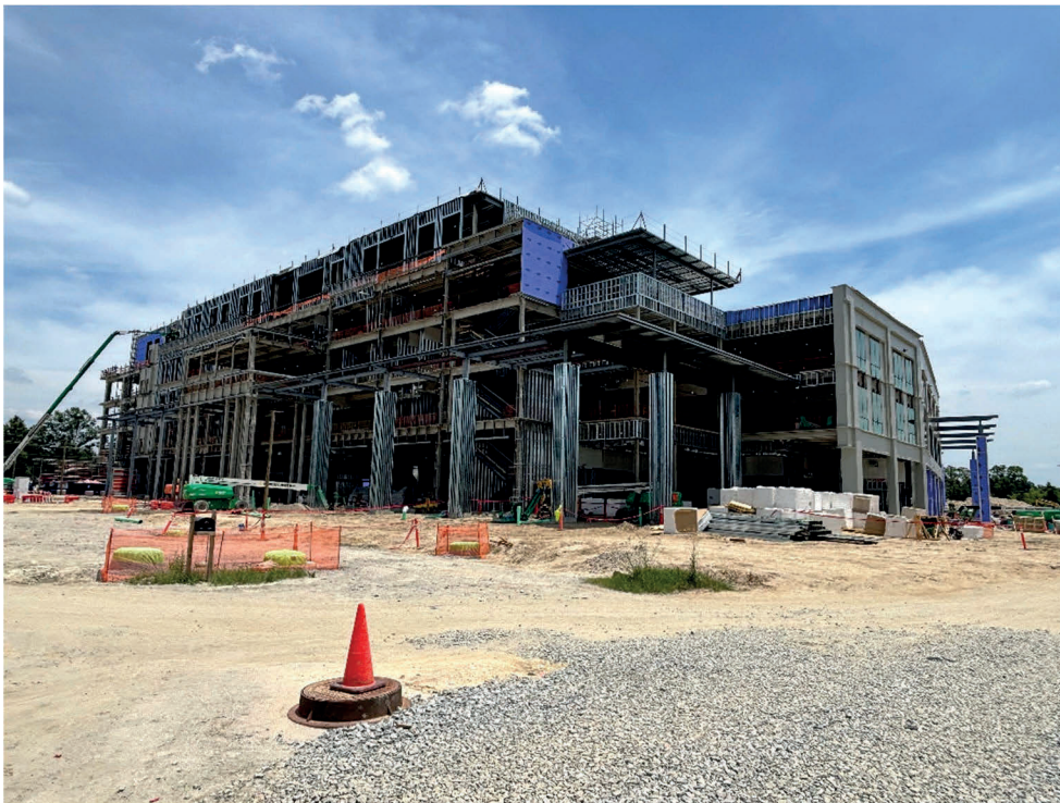
Photographs of the current School of Medicine Construction
