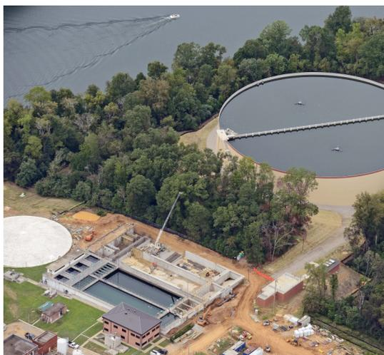
The City of North Augusta used \$26 million in SRF loans to construct a new, 30-million gallon raw water storage tank and raw water transfer pump station. Because of the loan, North Augusta officials were able to bring the system into compliance with state disinfection requirements and improve the system's reliability to protect the Savannah River, the system's raw water source.
