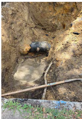
LEAD SERVICE LINES BEFORE REPLACEMENT
